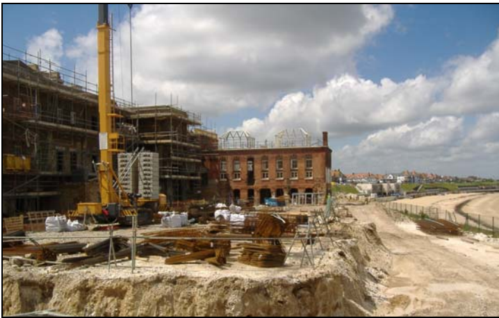
Construction work in progress on that part of Alexandra Court which faces the sea
